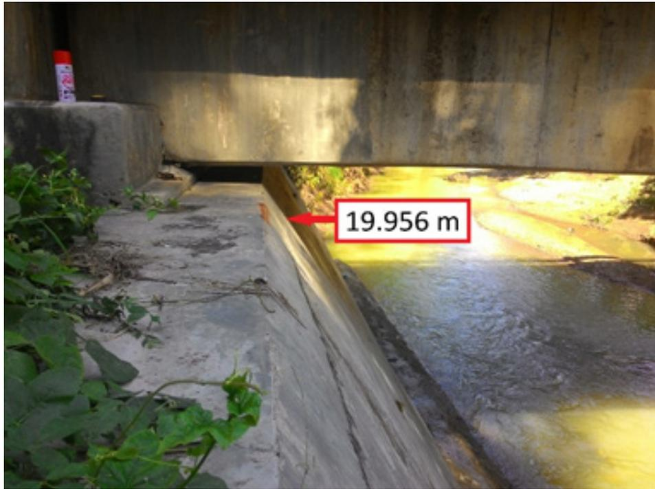
Figure 46. Water-level marking on an abutment of Cancahorao Bridge
