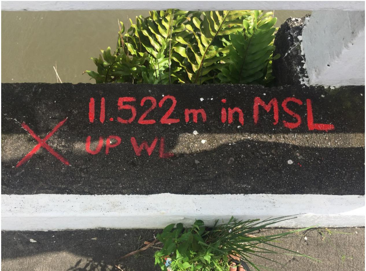
Figure 42. Water-level markings on Taboc Bridge
