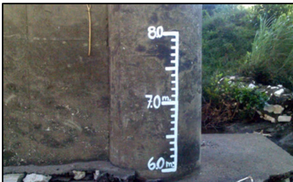
Figure 44. Water level markings on Baldoza Bridge
