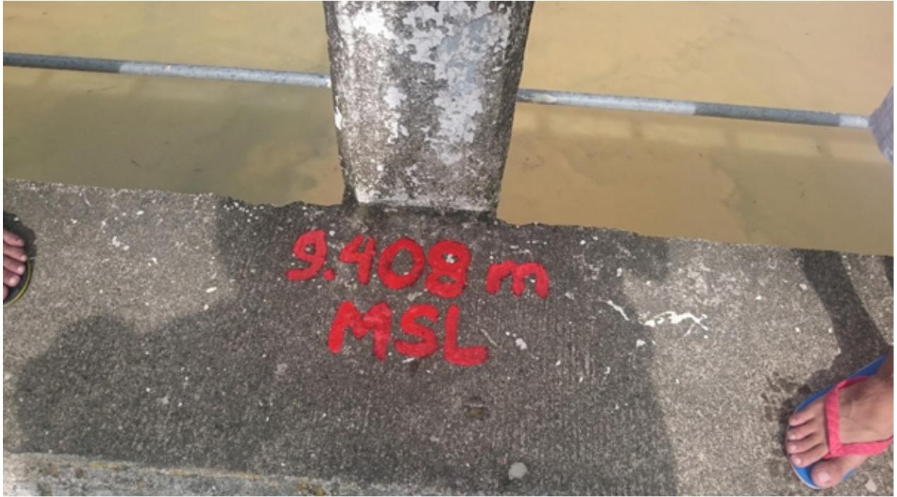
Figure 37. Water-level markings on Lagonoy Bridge
