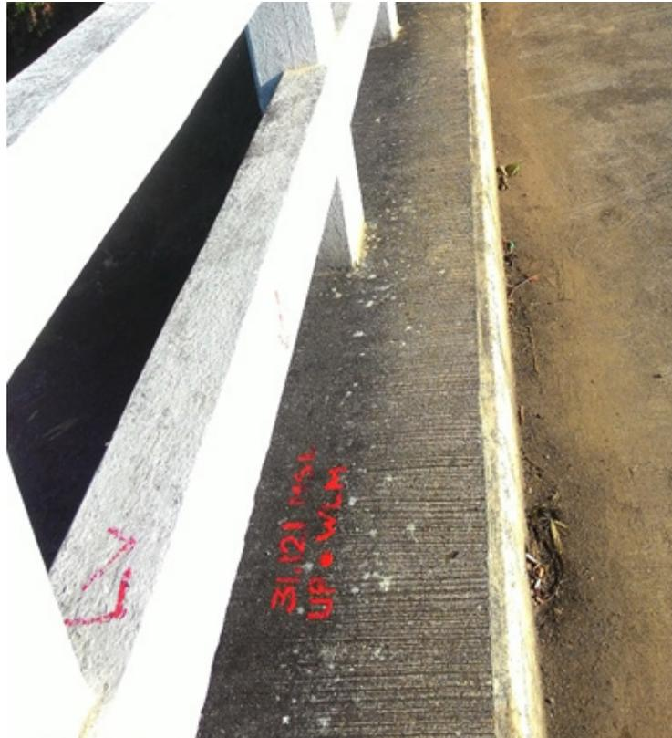
Figure 41. Water-level markings on the abutment of Lanang Bridge.
