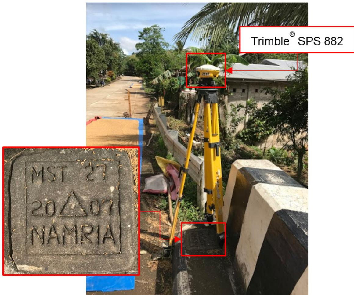
Figure 31. GNSS base set up, Trimble® SPS 882, at MST-27, located at the approach of Mabuaya Bridge in Brgy. Matiporon, Milagros, Masbate
