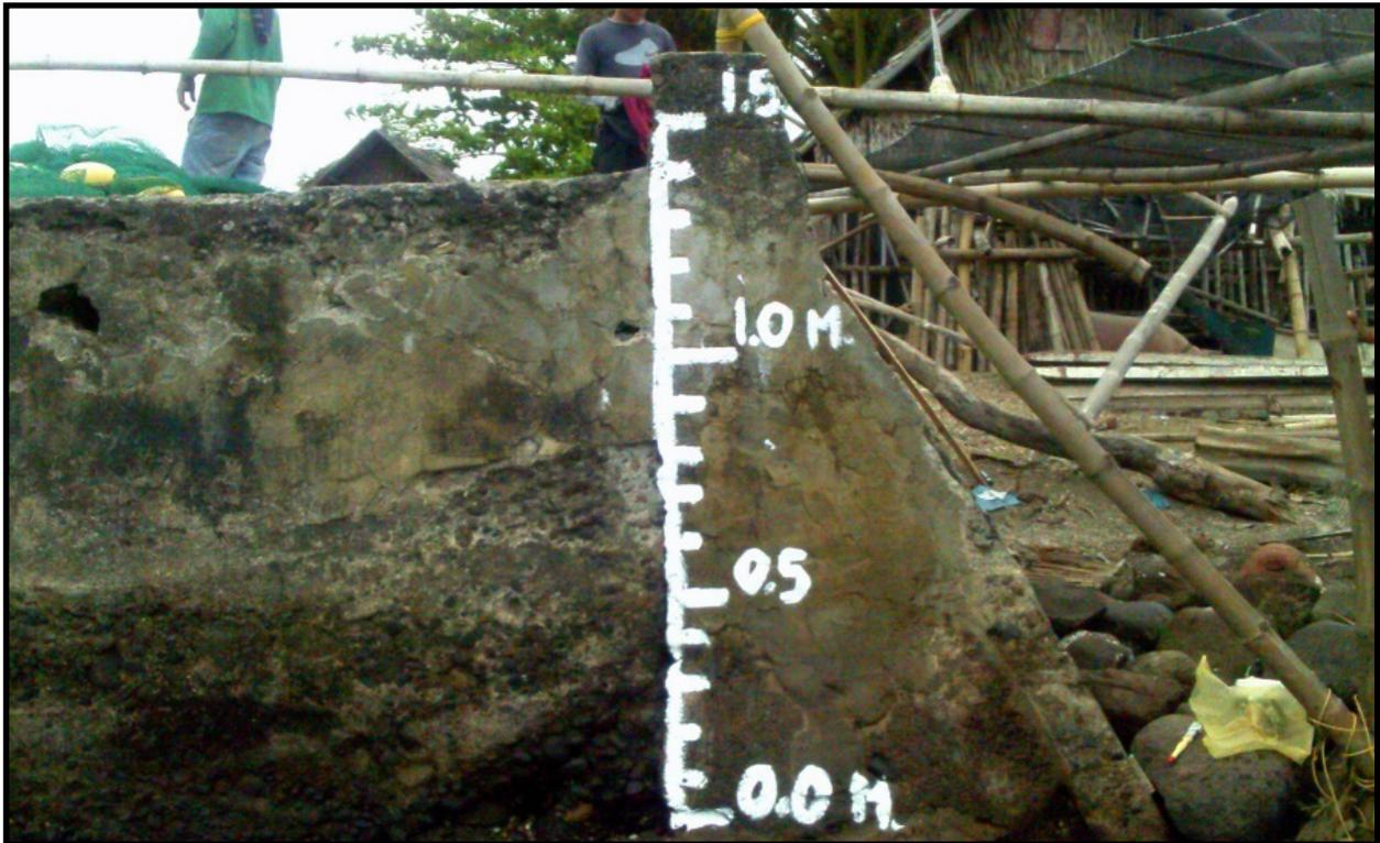
Figure 37. Water level markings at the side of the pier in Brgy. Bugtong, Mandaon, Masbate
