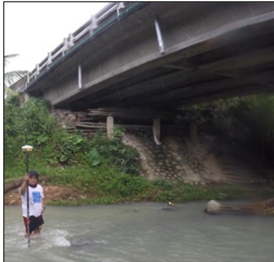
Figure 32. Cross-section and bridge as-built survey for Batu Bridge, Brgy. Batu, Zamboanga Sibugay
