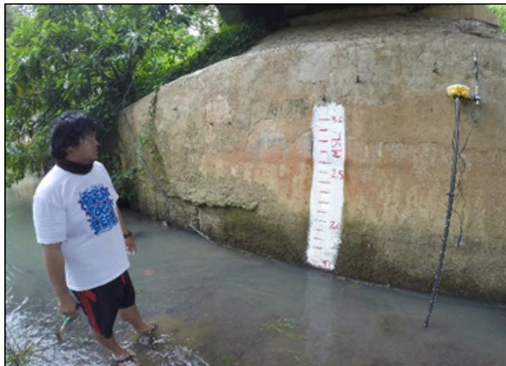
Figure 36. Water level markings on the post of Batu Bridge.
