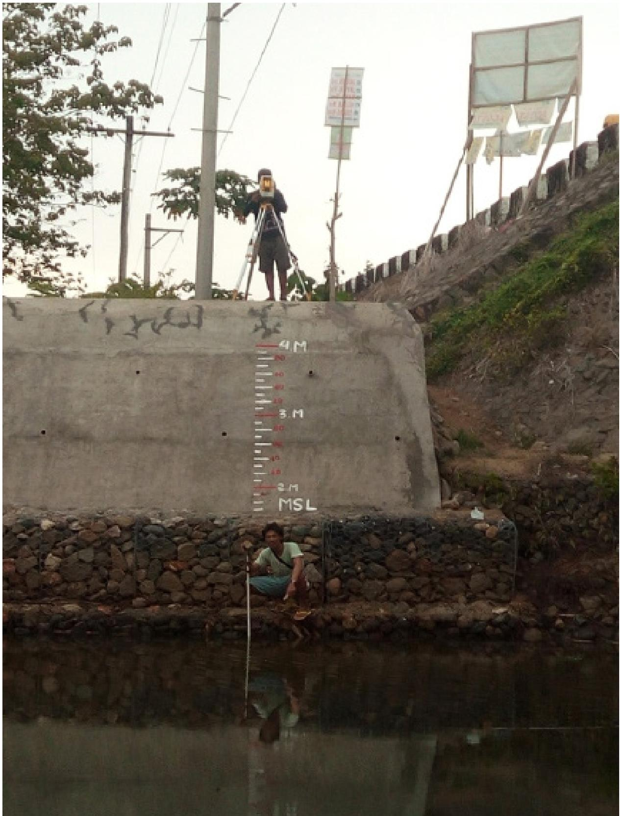
Figure 40. Water-level markings on Buluan Bridge
