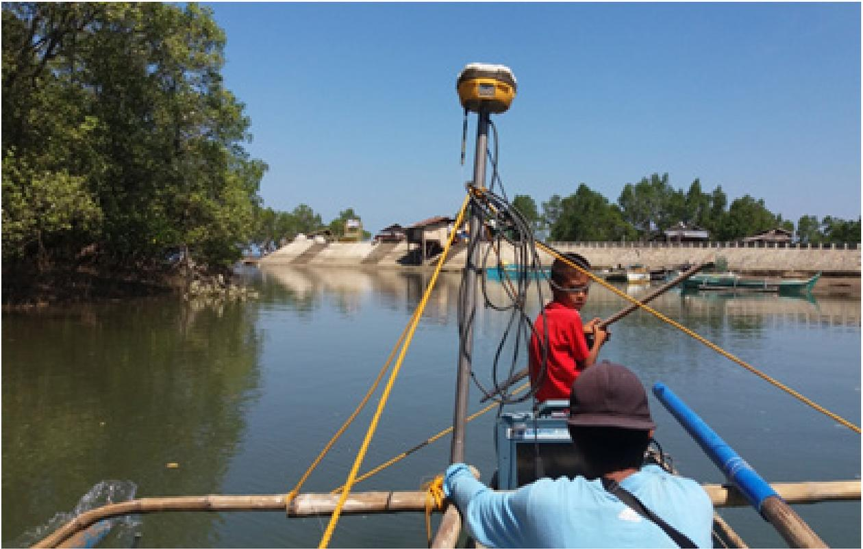
Figure 44. Bathymetric survey of ABSD at Buluan (also known as Digsa) River using Hi-Target™ Echo Sounder (upstream)
