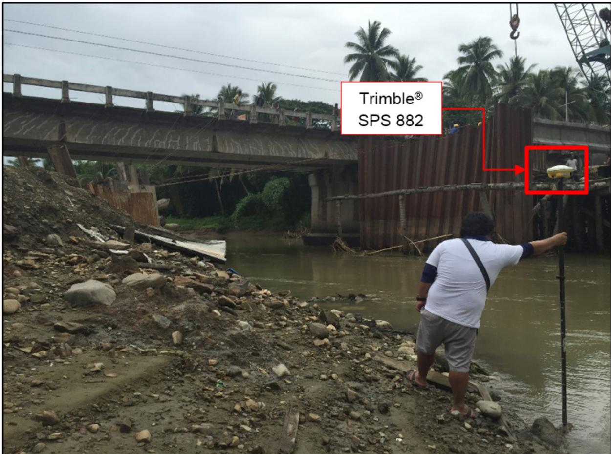
Figure 34. Cross-section and bridge as-built survey for Kabasalan Bridge, Brgy.Sininan, Municipality of Kabasalan. The construction of the new bridge is ongoing.
