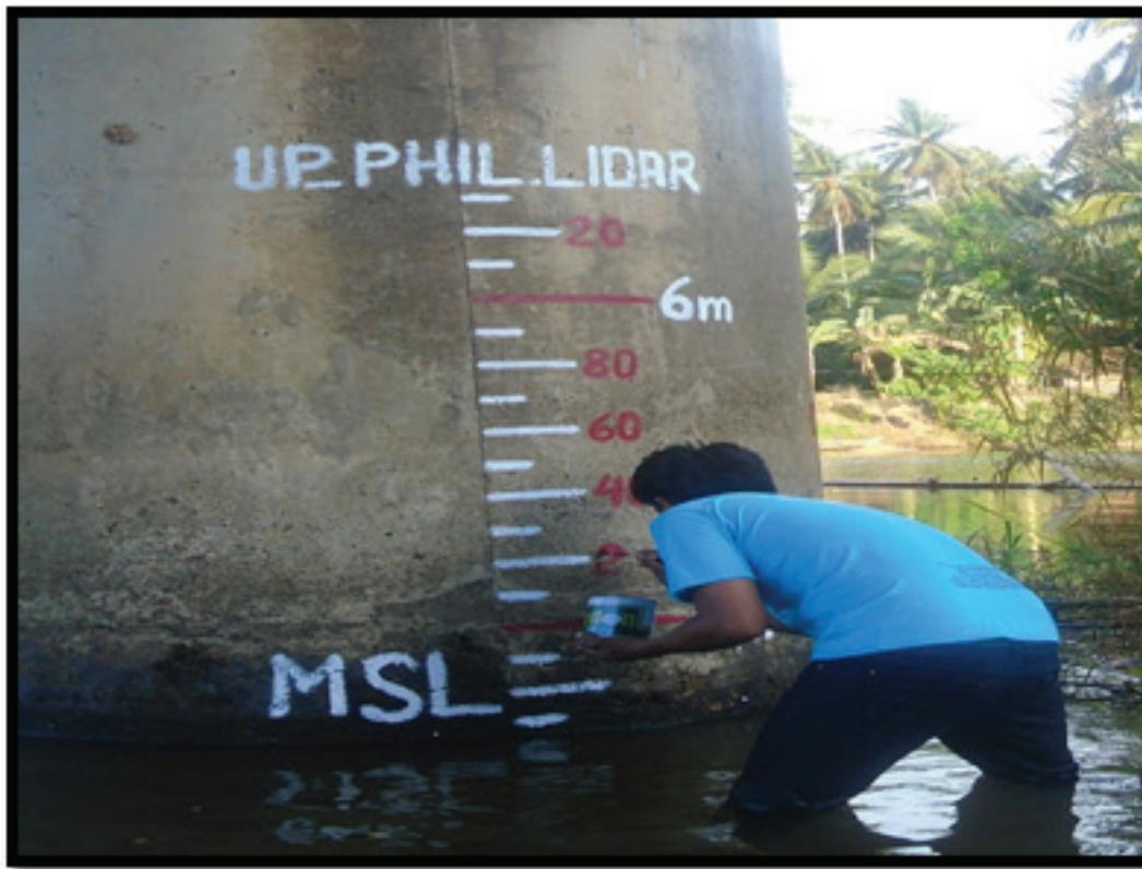
Figure 38. Water-level markings on Kipit Bridge
