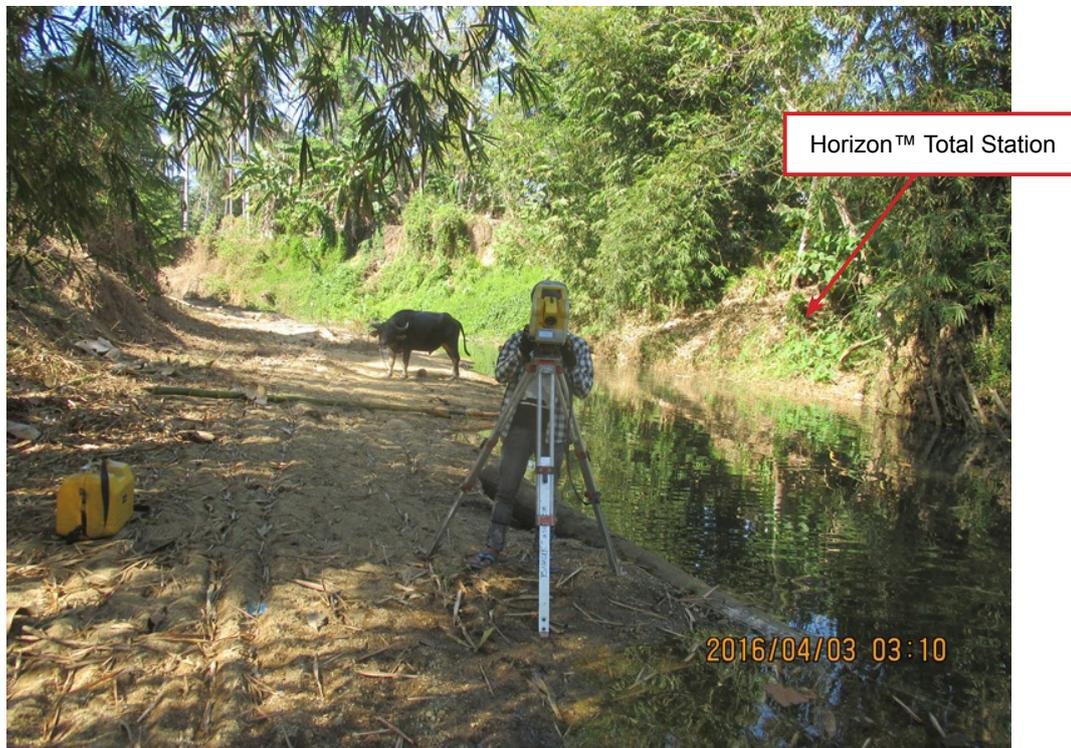
Figure 44. Bathymetric survey at Labason River using a Horizon™ Total Station
