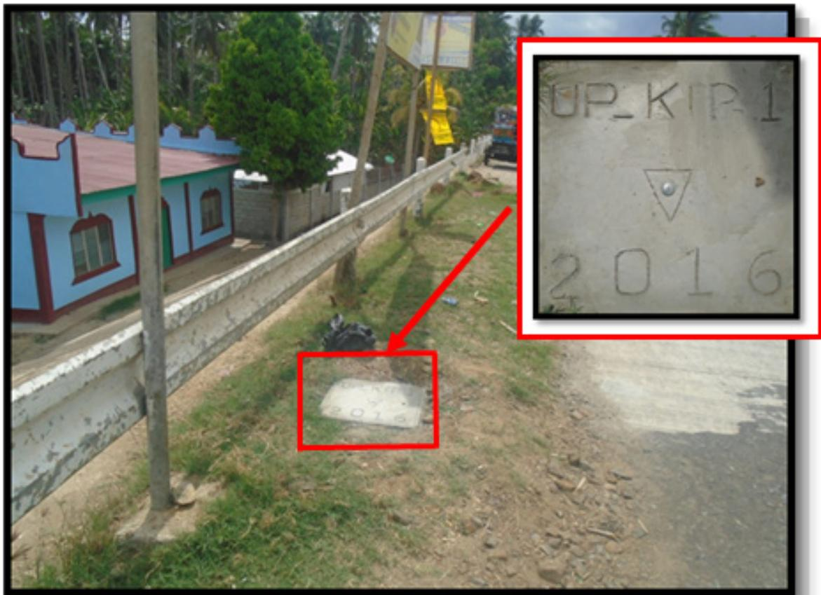
Figure 32. UP\_KIP-1 located at the approach of Kipit Bridge in Brgy. Kipit, Municipality of Labason, Province of Zamboanga del Norte
