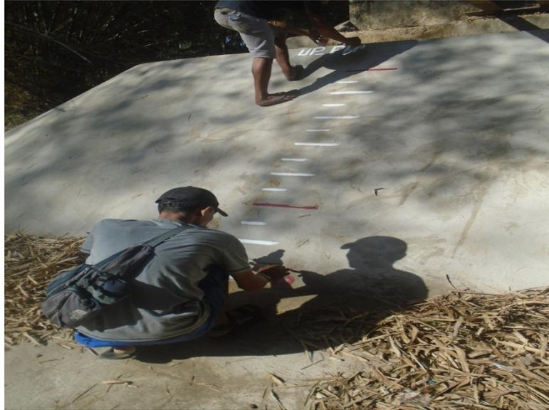
Figure 41. Water-level markings on Labason Bridge
