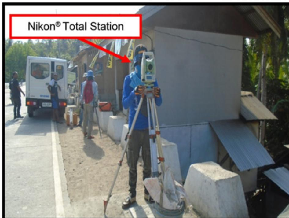
Figure 36. As-built survey of Patawag Bridge
