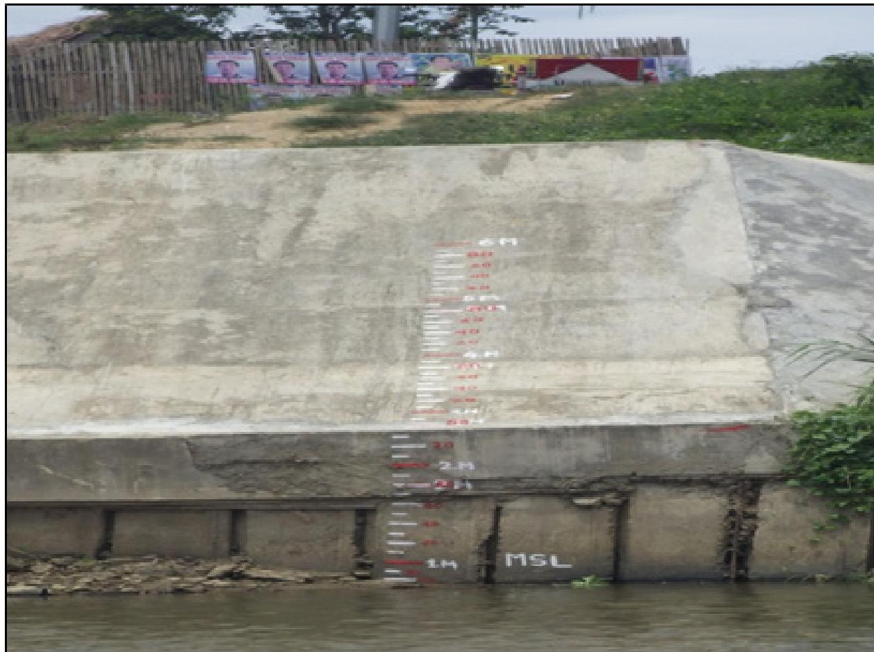
Figure 40. Water-level markings on Siocon Bridge
