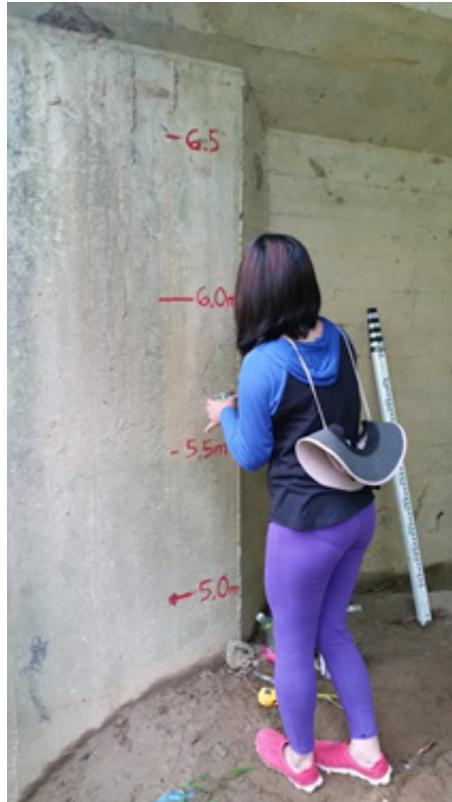
Figure 46. Water-level marking at Vitali Bridge's Footing.
