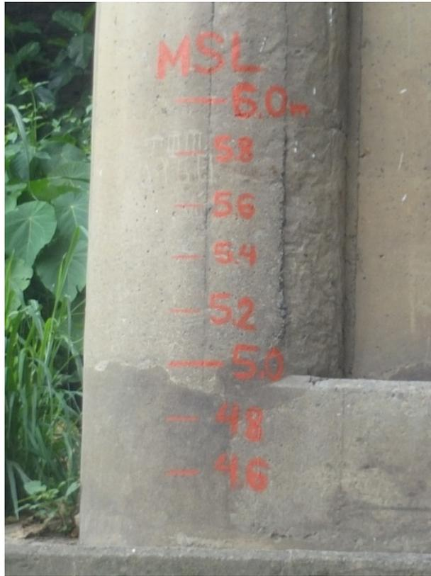
Figure 41. Water-level markings on Talisay Bridge
