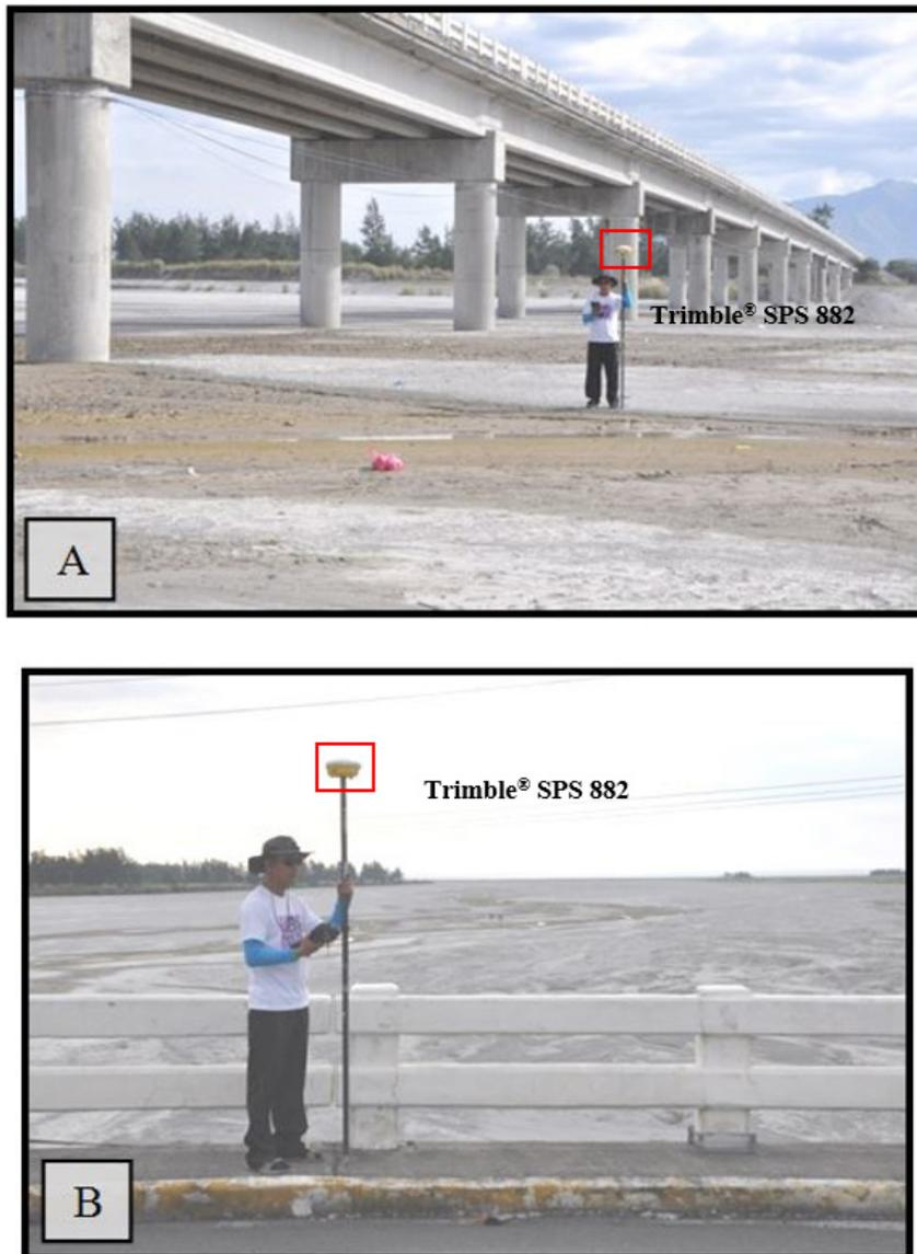
Figure 36. (A) Bridge as-built survey and (B) cross-section survey in Maculcol Bridge, Municipality of San Narciso
