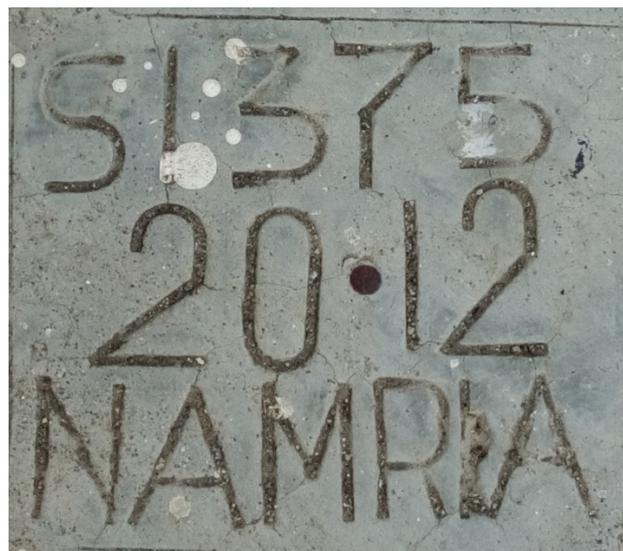
Figure 31. SI-375, a NAMRIA established BM, located along the national highway in Brgy. Kabatiol, Maasim, Sarangani
