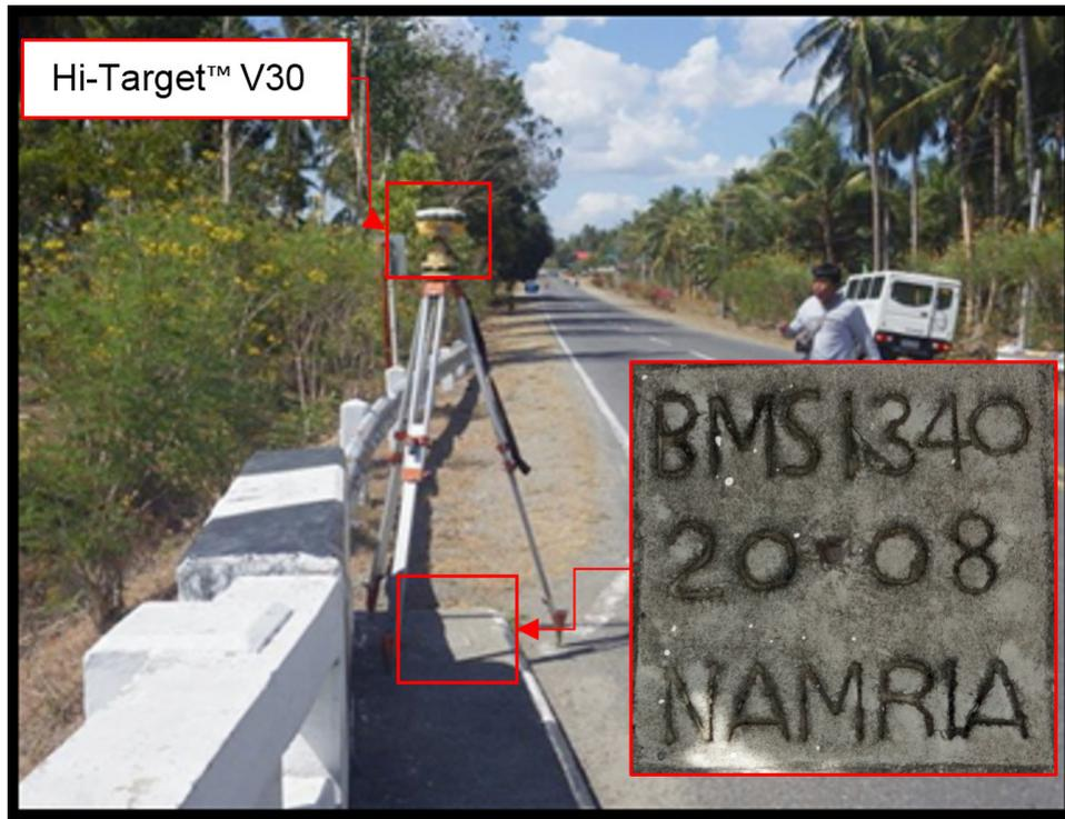
Figure 30. GNSS receiver set up, Hi-Target™ V30, at BMSI-340, located at the approach of Molo Bridge in Brgy. Lun Masla, Malapatan, Sarangani
