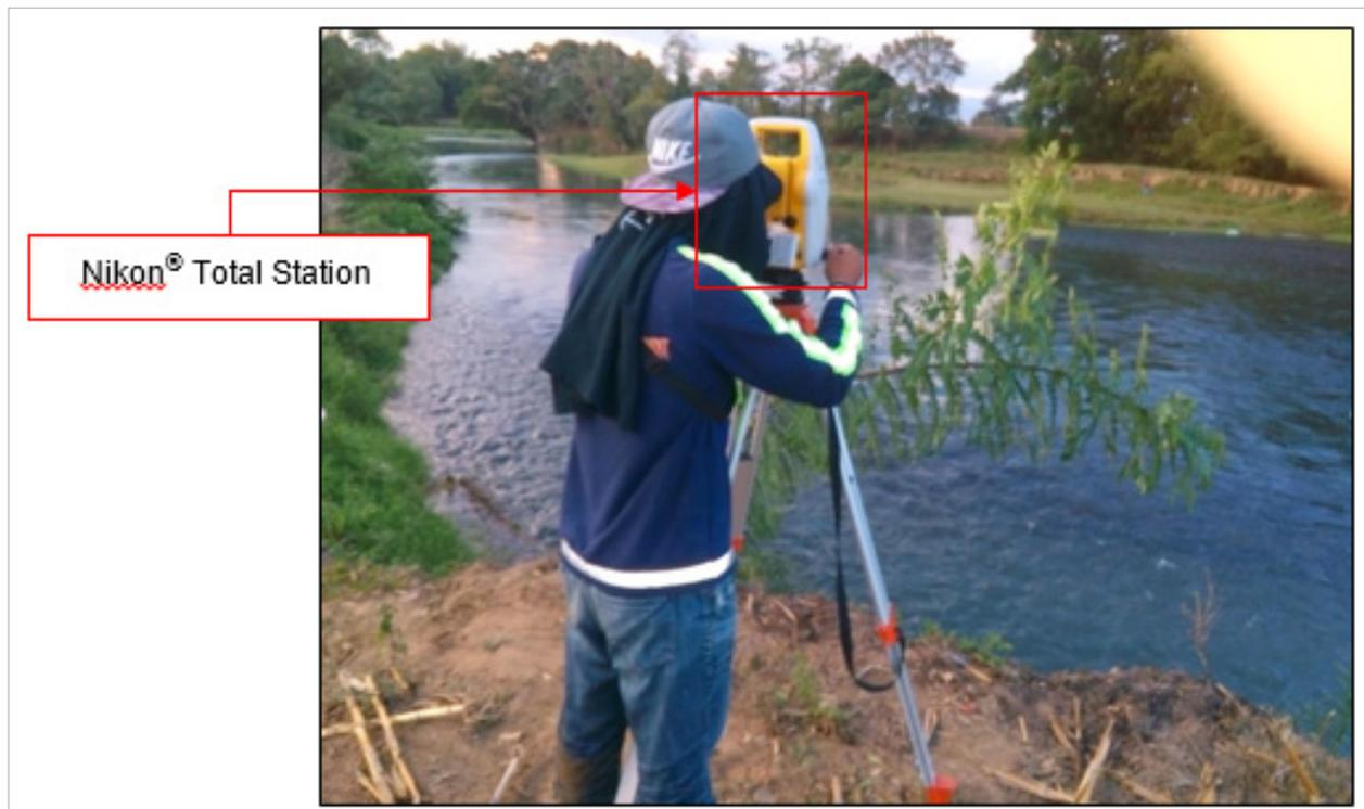
Figure 46. Manual Bathymetric survey of ABSD at Manupali River using Nikon® Total Station
