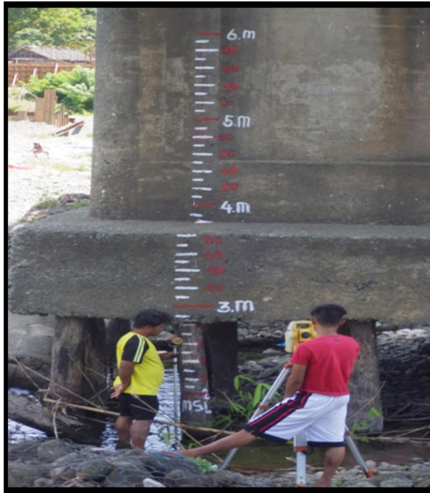
Figure 38. Water-level markings on Magallanes Bridge
