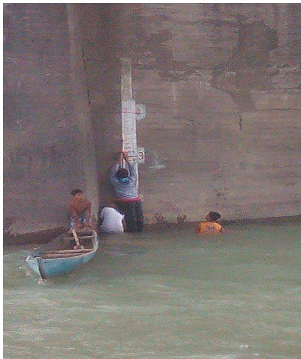
Figure 45.Water level markings on the post of Abulug Bridge
