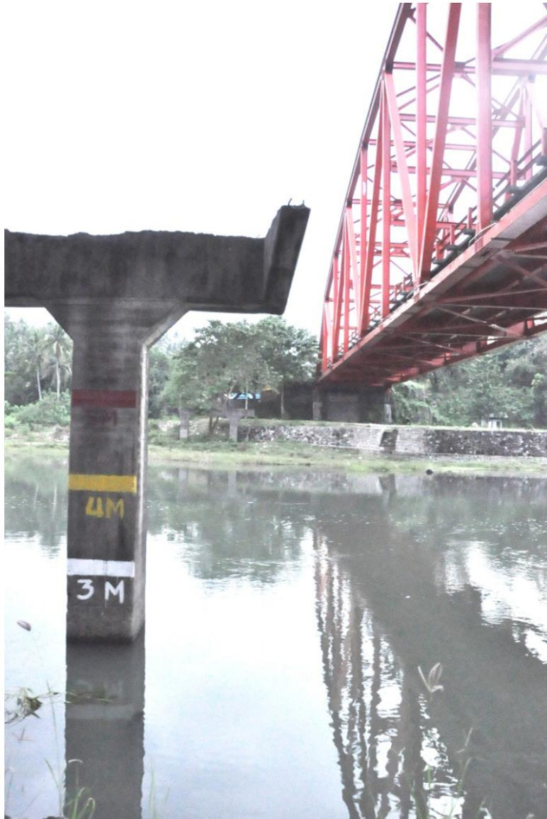
Figure 40. Water level mark at one of the piers of the old Pateng Bridge
