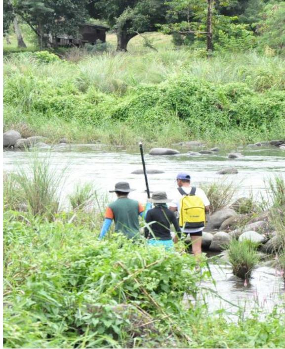
Figure 44. Team A performing manual bathymetric survey going upstream of Aunugay River
