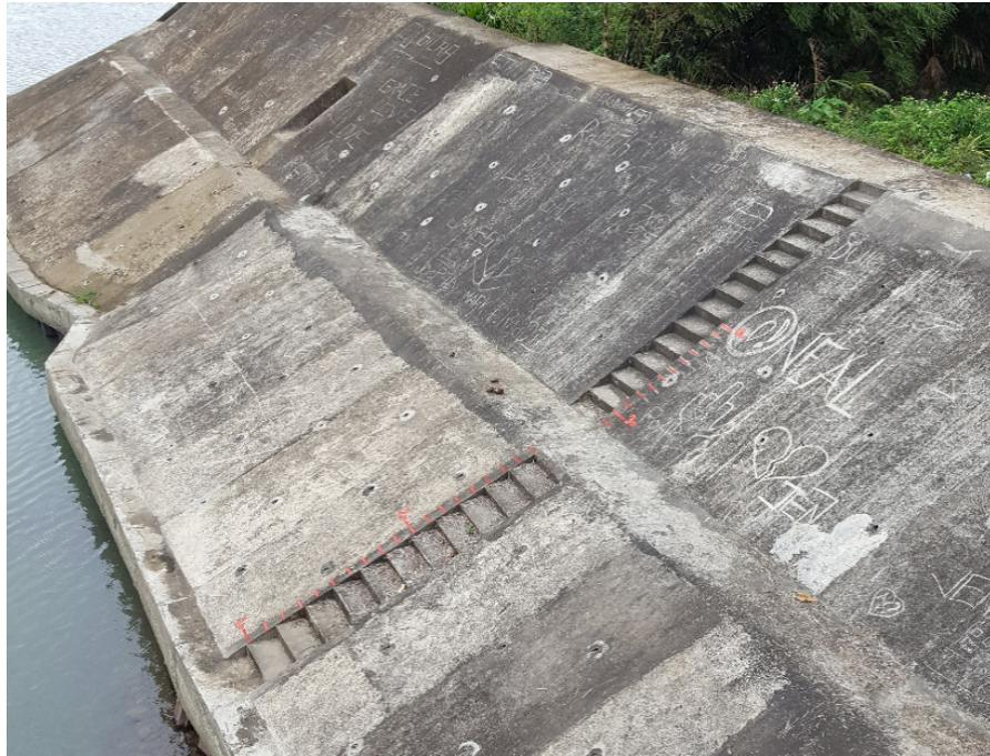
Figure 44. Water level markings on the riprap of Baua Bridge
