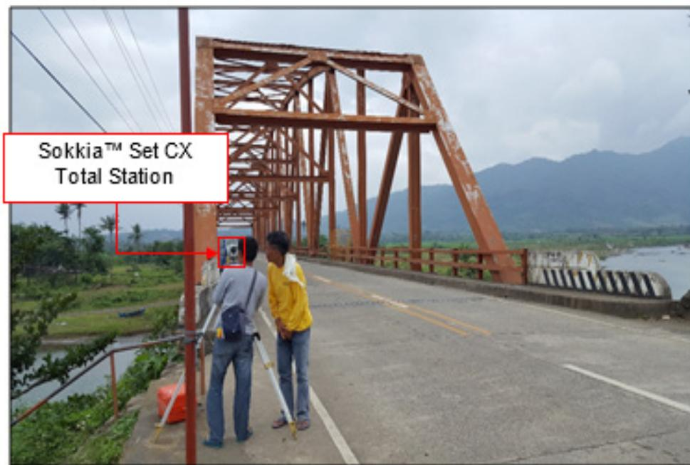
Figure 39. As-built survey of Baua Bridge
