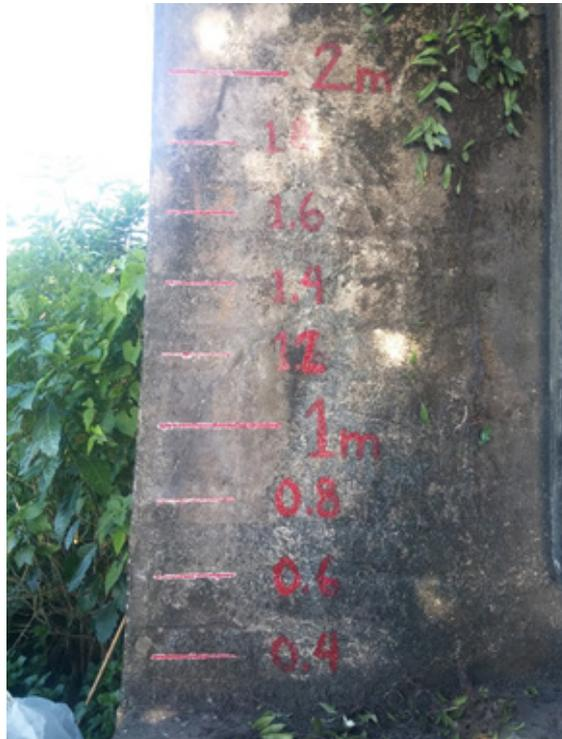
Figure 41. Water-level markings on the Cabcungan Bridge
