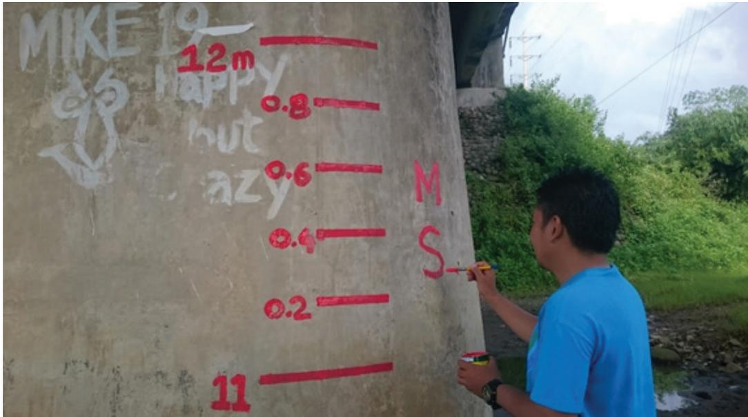
Figure 38. Water-level markings on Casambalangan Bridge
