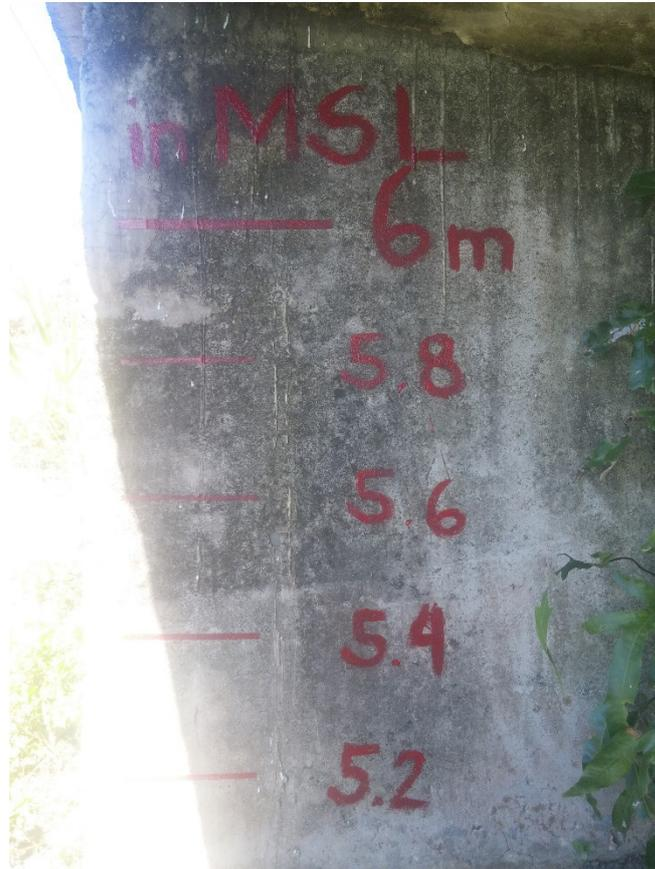
Figure 44. Water-level markings on the Linao Bridge
