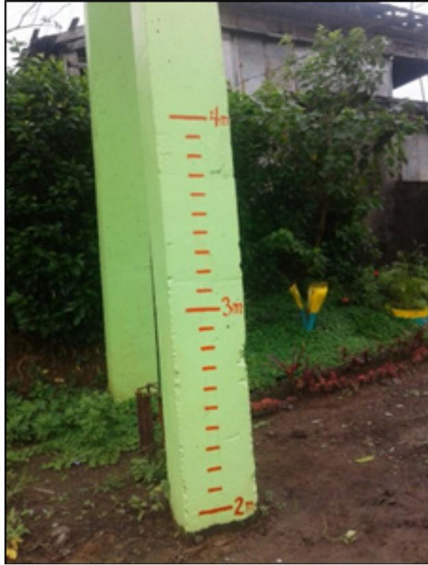
Figure 41. Water level markings on the post of Casagan Hanging Bridge
