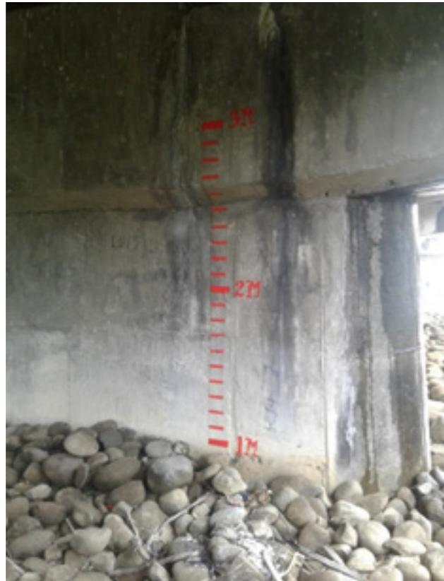
Figure 42. Water level marking on the pier of Sta. Cruz Bridge
