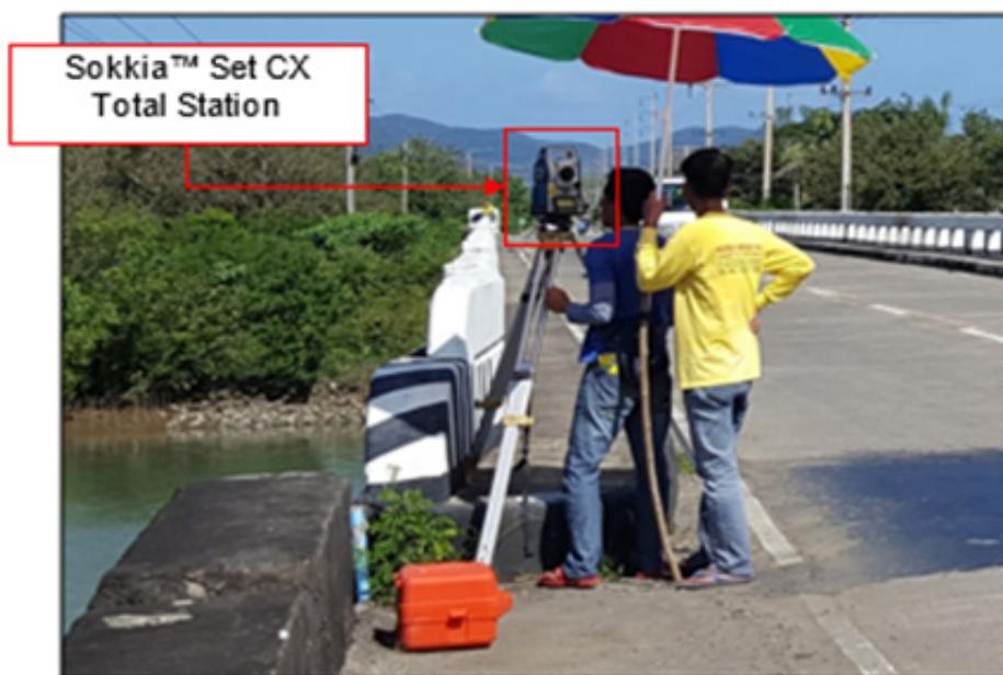
Figure 36. As-built survey of Sta. Cruz Bridge
