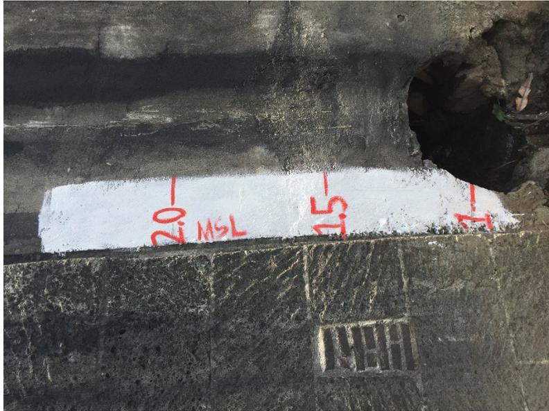
Figure 43. Water level markings on the side of the pier of the Zapote Bridge
