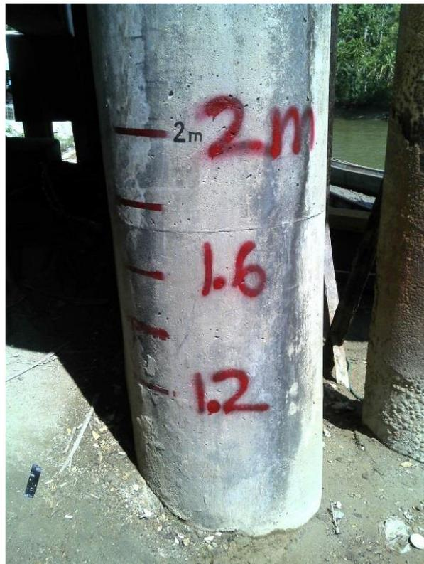
Figure 45. Painting of water level markings on Calauag Bridge
