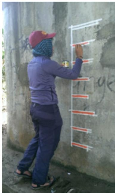
Figure 39. Water Level Marking for Catanauan River.
