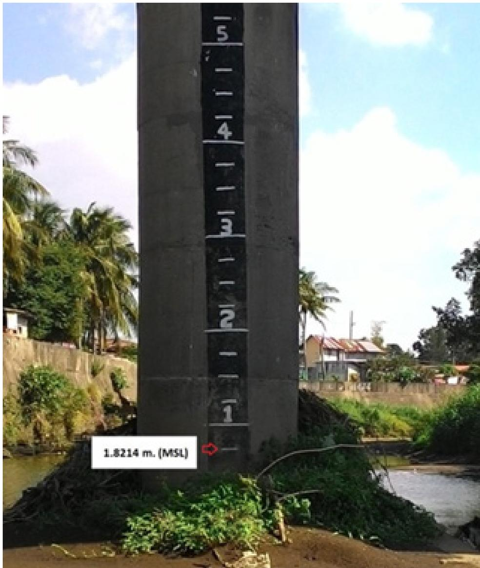
Figure 41. Existing bridge marking and the corresponding MSL elevation.
