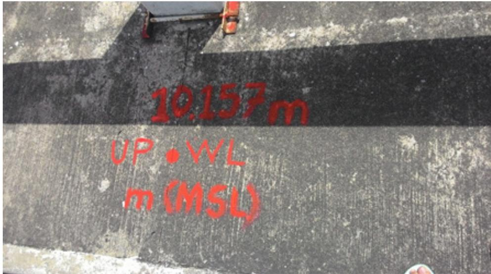
Figure 37. Water-level markings on Kilbay Bridge.
