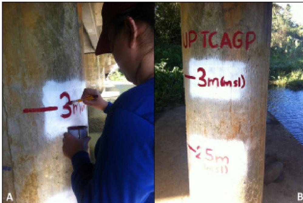
Figure 36. (A) Actual water-level marking on Lubayat Bridge and (B) finished markings on the bridge pier
