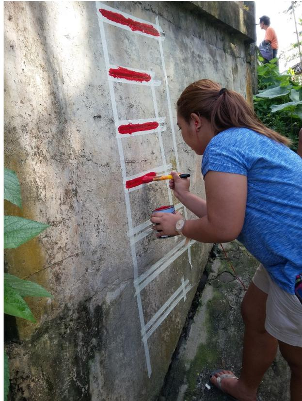
Figure 46. Water-Level Markings on Macalelon Bridge
