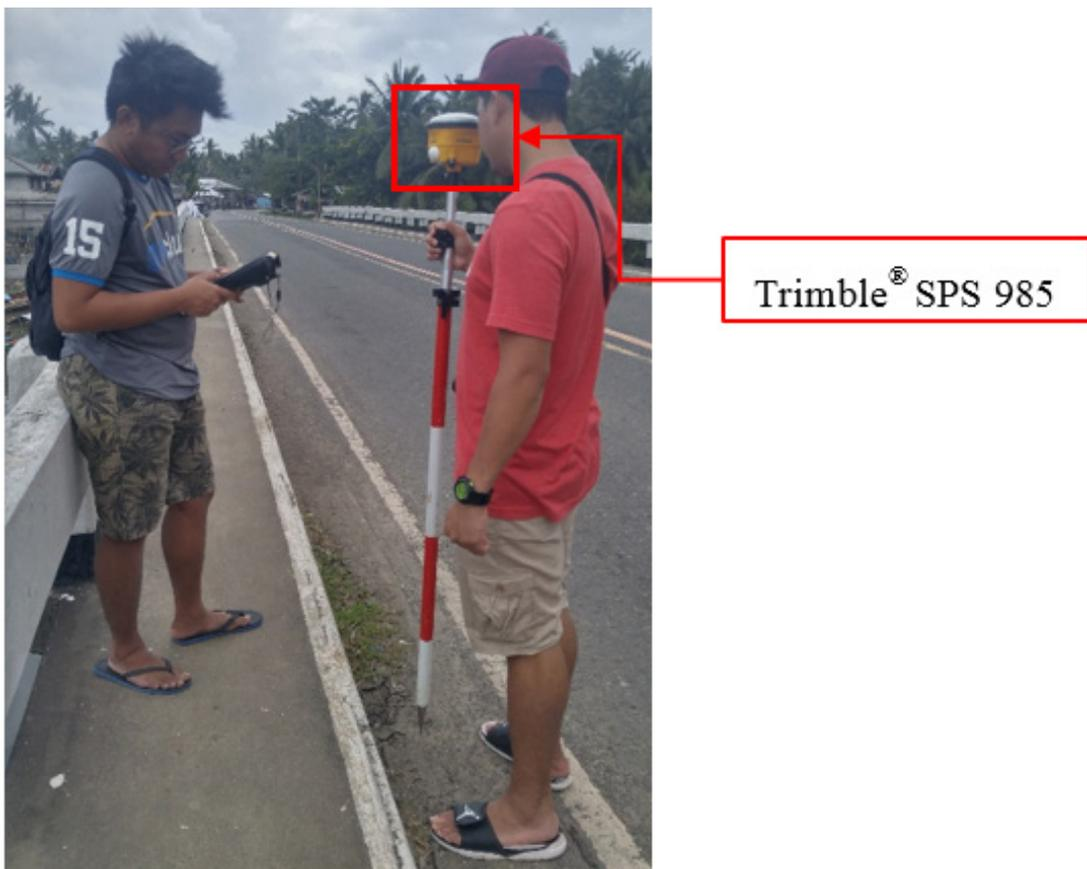
Figure 42. Bridge As-Built Survey using PPK Technique.
