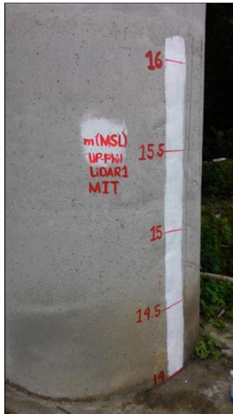
Figure 41. Water level markings on the side of the pier of the Mabacao Bridge
