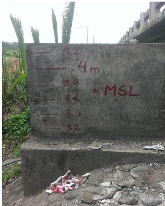
Figure 45. Mean Sea Level (MSL) elevation markings for Pandanan River
