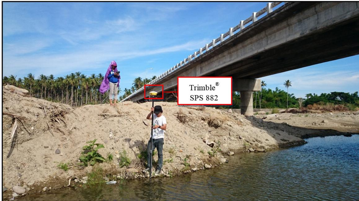
Figure 35. Cross-section survey conducted on Rosario-Lobo River in Brgy. Lagadlarin, Municipality of Lobo
