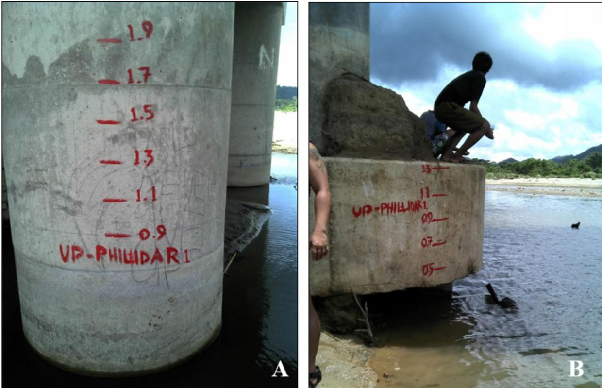
Figure 38. Marking of MSL-based elevation on the pier on the left side facing downstream (A) and right side (B) at the Lobo Bridge, Lobo Batangas
