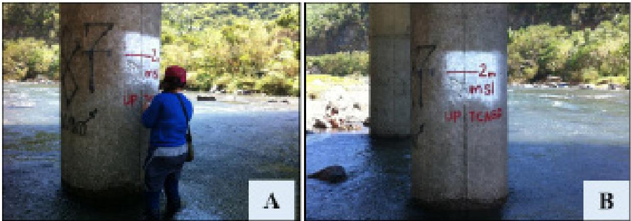
Figure 37. MSL water level markings in Tignoan Bridge's pier
