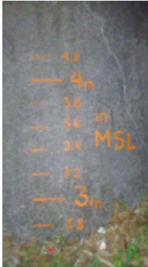
Figure 45. Water-level markings on New Vigo Bridge
