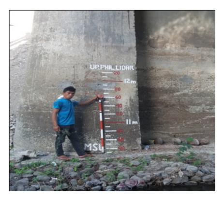
Figure 48. Water-level markings on Balili Bridge
