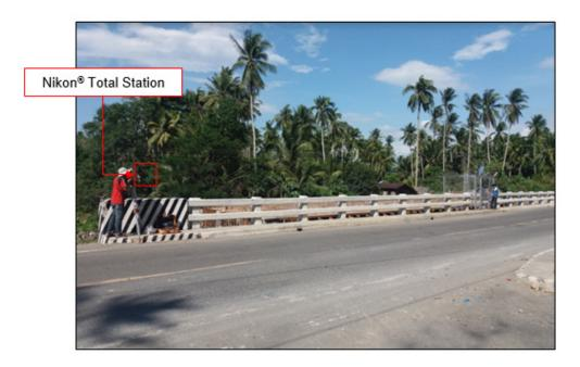
Figure 44. As-built survey of Balili Bridge
