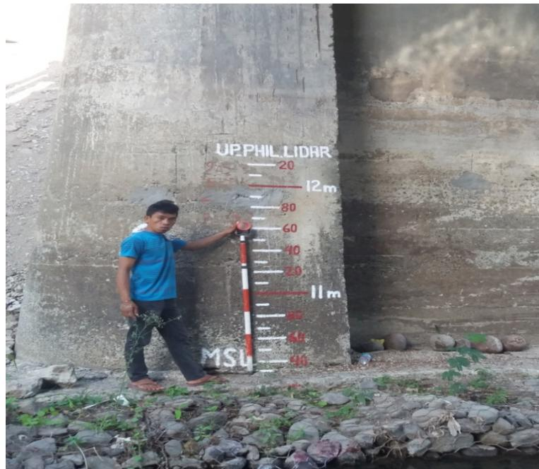
Figure 48. Water-level markings on the Butadon Bridge
