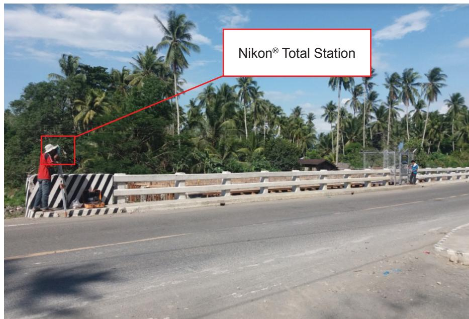
Figure 44. As-built survey of Butadon Bridge
