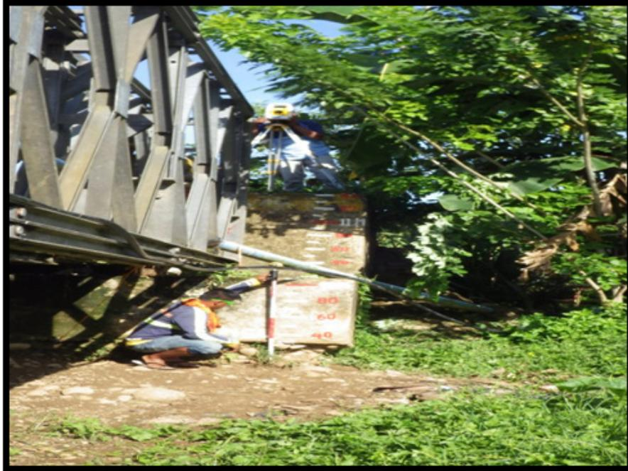
Figure 41. Water-level markings on Kumalarang (Boyugan East) Bridge
