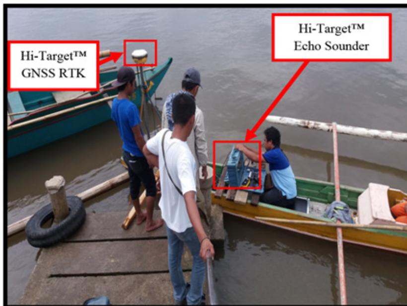
Figure 44. Bathymetric survey of ABSD at Kumalarang River using Hi-Target™ Echo Sounder (upstream)
