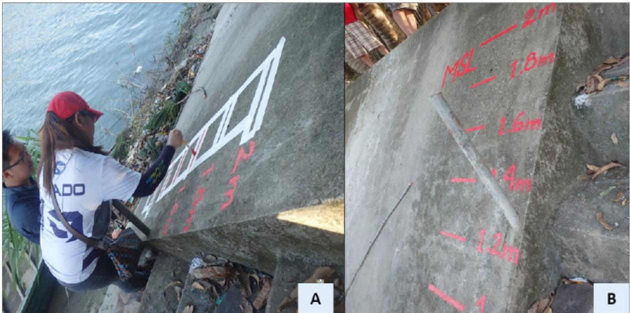
Figure 46. MSL water level markings at Labangan Bridge's Abutment
