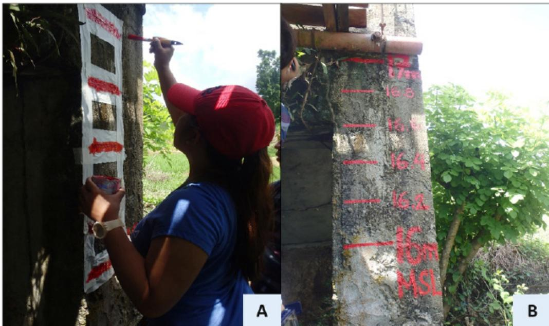
Figure 47. MSL water level markings at Hanging Bridge's Foot
