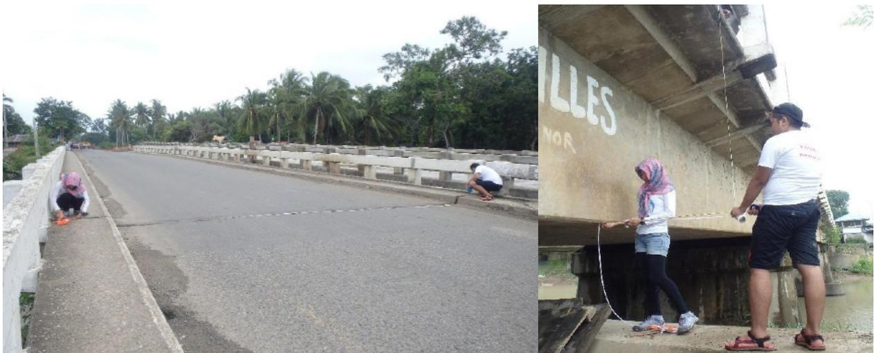
Figure 39. As-built survey at Labangan Bridge in Brgy. New Labangan, Labangan, Zamboanga del Sur
