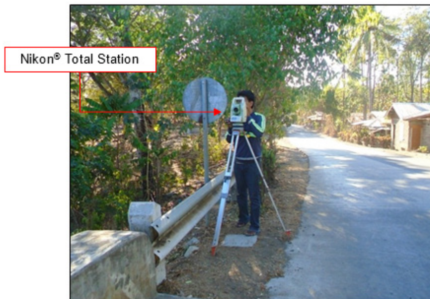
Figure 39. As-built survey of the Calabayan Bridge
