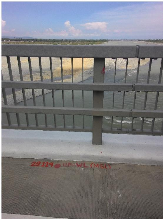
Figure 38. Water-level markings on the deck of Amburayan Bridge.
