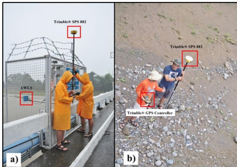
Figure 40. a) Getting the elevation of an installed AWLS during as-built survey and b) cross-section survey along the downstream side of Cabaroan Bridge after the river water has subsided
