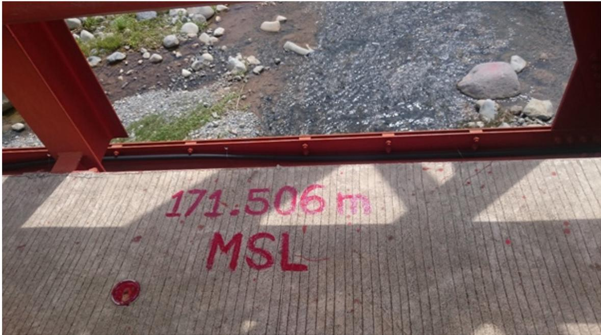
Figure 59. Water-level markings on Manicbel Bridge
