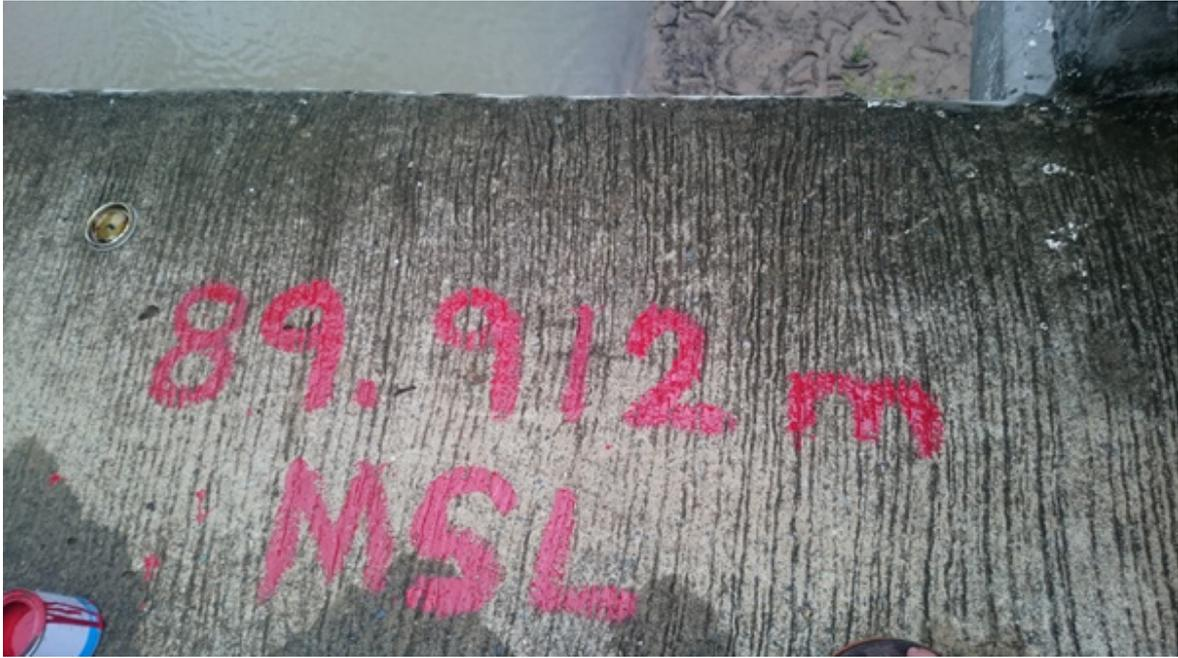
Figure 57. Water-level markings on Cervantes Bridge
