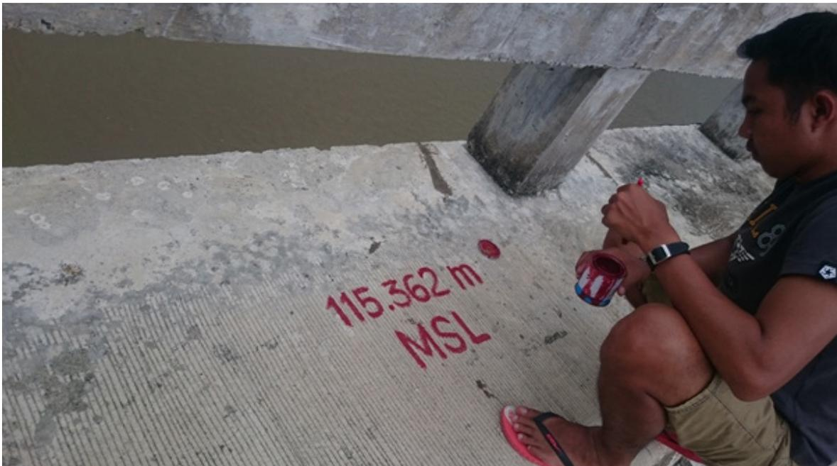
Figure 58. Water-level markings on Manabo Bridge
