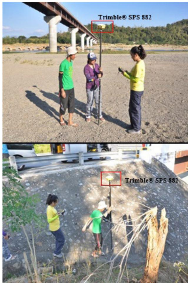
Figure 34.(a) Cross-Section survey at Sarrat Bridge and (b) conduct of the bridge as-built survey
