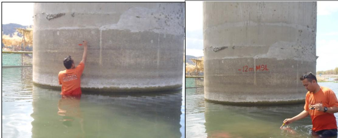
Figure 39. Water Level Marking for Sarrat Bridge
