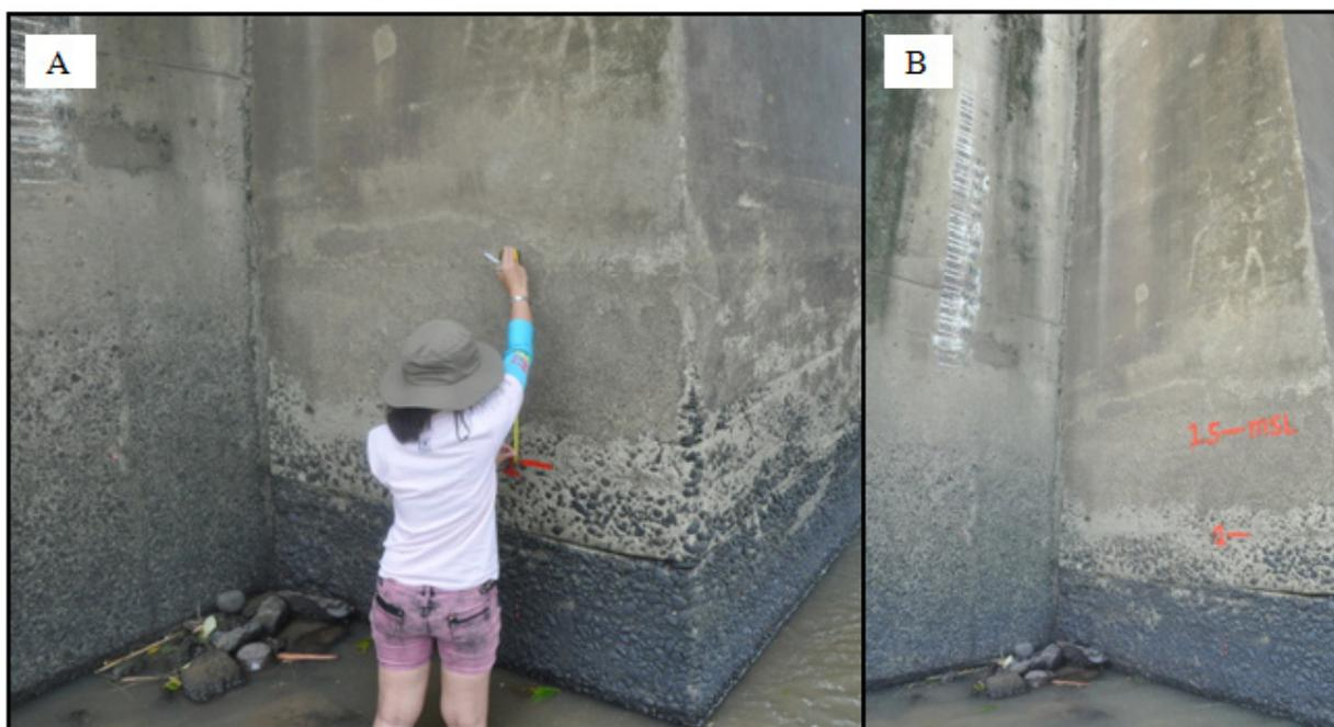
Figure 38. (A) Marking of bridge pier and (B) Water Level Mark at the pier of Troso Bridge
