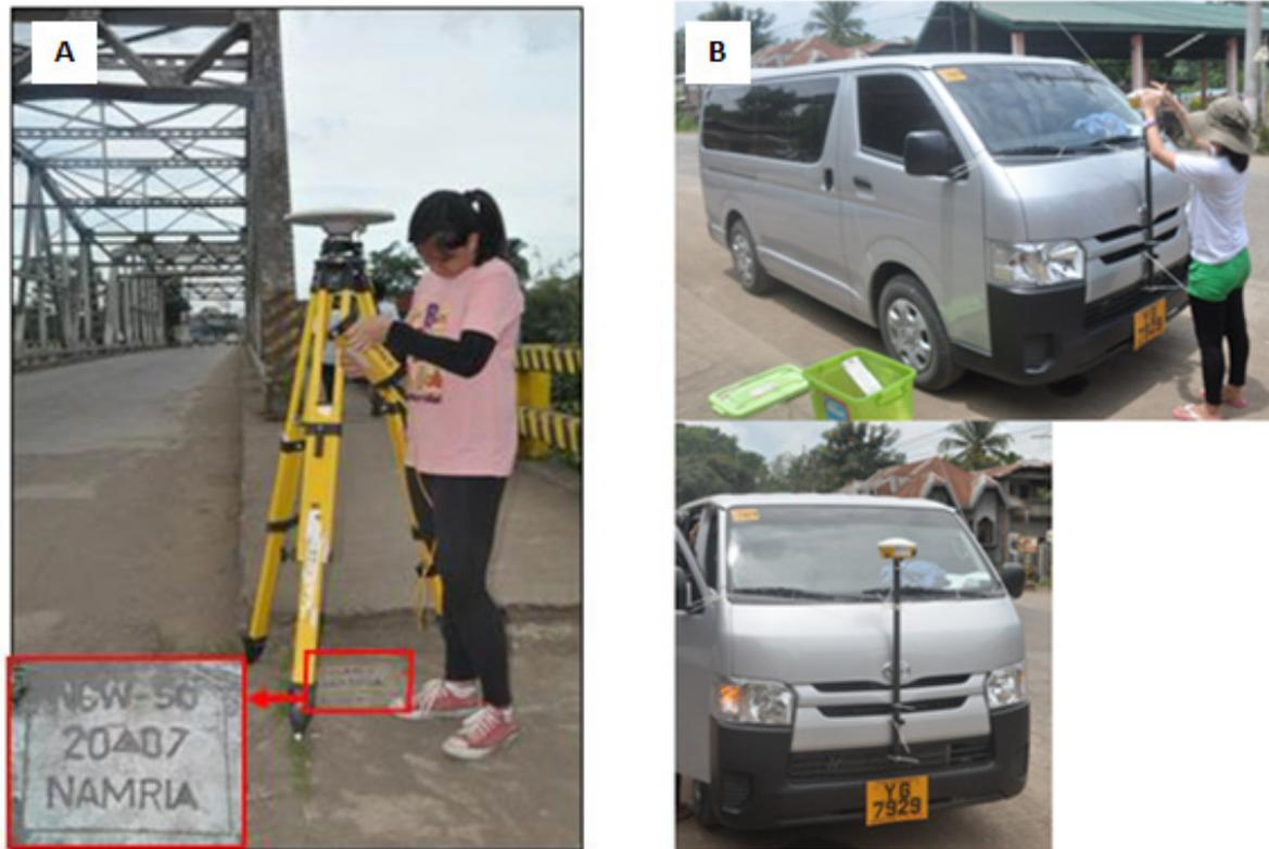
Figure 42. (A) Occupied base station, NGW-50 in Himogaan Bridge, Sagay City and (B) Installation of GNSS Receiver Trimble® SPS 882 in front of a van
