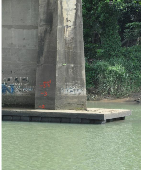
Figure 41. Water Level Mark at the pier of Himogaan Bridge
