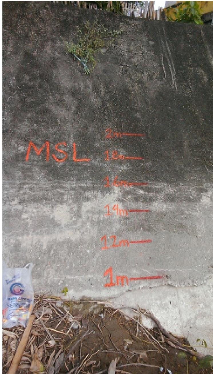
Figure 38. Painting of water level markings on Ibajay Bridge.
